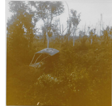
13 Rome Plow.JPG | A good part of my time in the 25th saw my unit providing security for Rome Plows (pictured here) that were pretty much clearing areas to eliminate any possibility of enemy concealment. These plows were similar to bulldozers and were actually made by the Rome Plow Company in Georgia. (1136x1152)
